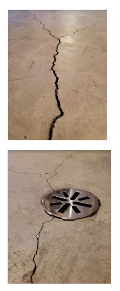
The air pressure inside your home is usually lower than in the soil surrounding the foundation. This difference in pressure draws air and other gases, including radon, from the soil into your home.
